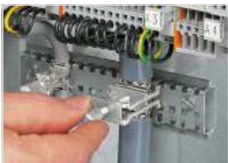
Tightening/removing a shield clamping saddle.
