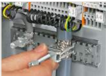
Securing an additional shield clamping saddle.
