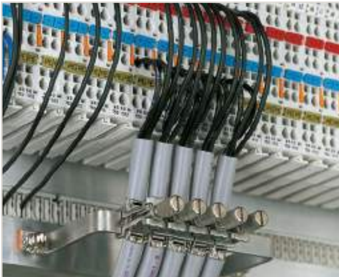
U-shaped (10 x 3) mm copper busbar
